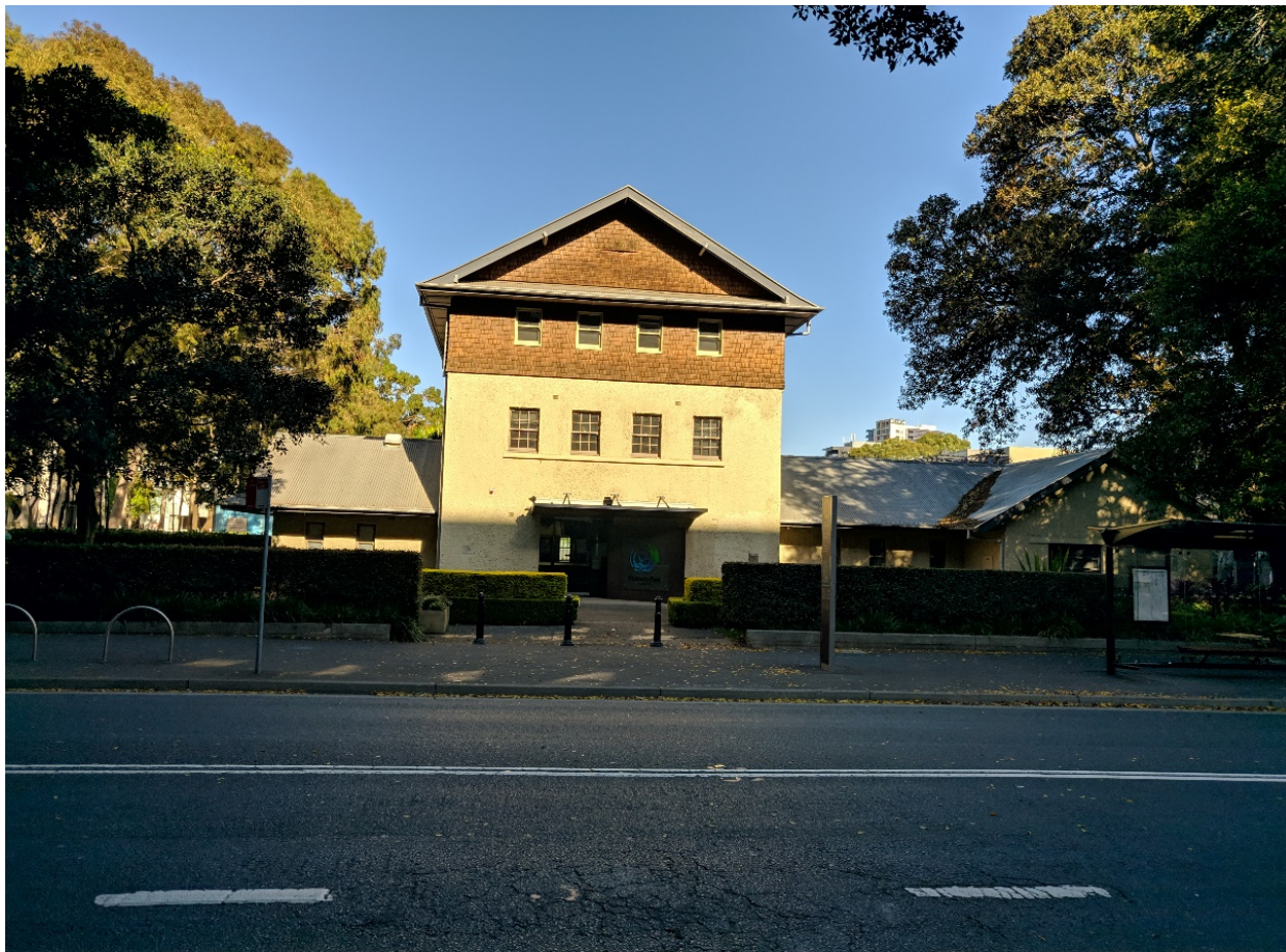
Joynton Avenue frontage
